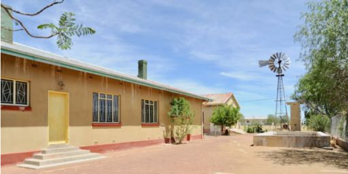
Two adjoining properties were secured by the Wolwedans Foundation in 2021 to form the ‘home’ and logistical base of the project. The properties will house the Laundry, Greenhouses and the initial Barn as well as project staff accommodation.
