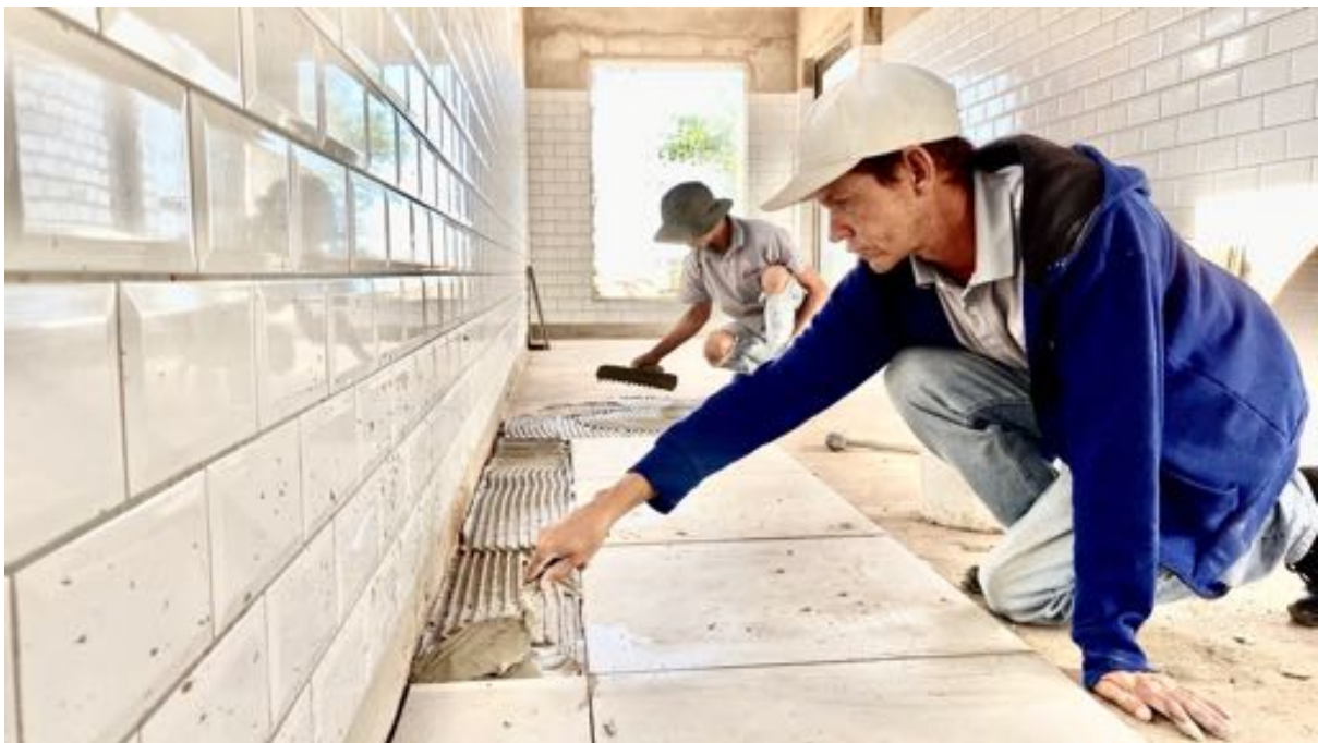
A special bottling room was built close to the pump house in 2021 to house the bottling plant in a hygienic environment.
