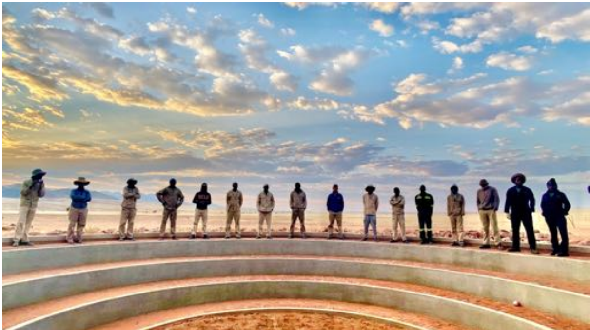
The morning circle (completed in Feb 2021) serves both as a daily assembly point for team, trainees, contractors and visitors alike, as well as a cultural event and performing arts venue. It brings people together each morning - on the periphery of Wolwedans Village, creating a wonderful sense of community and togetherness.
