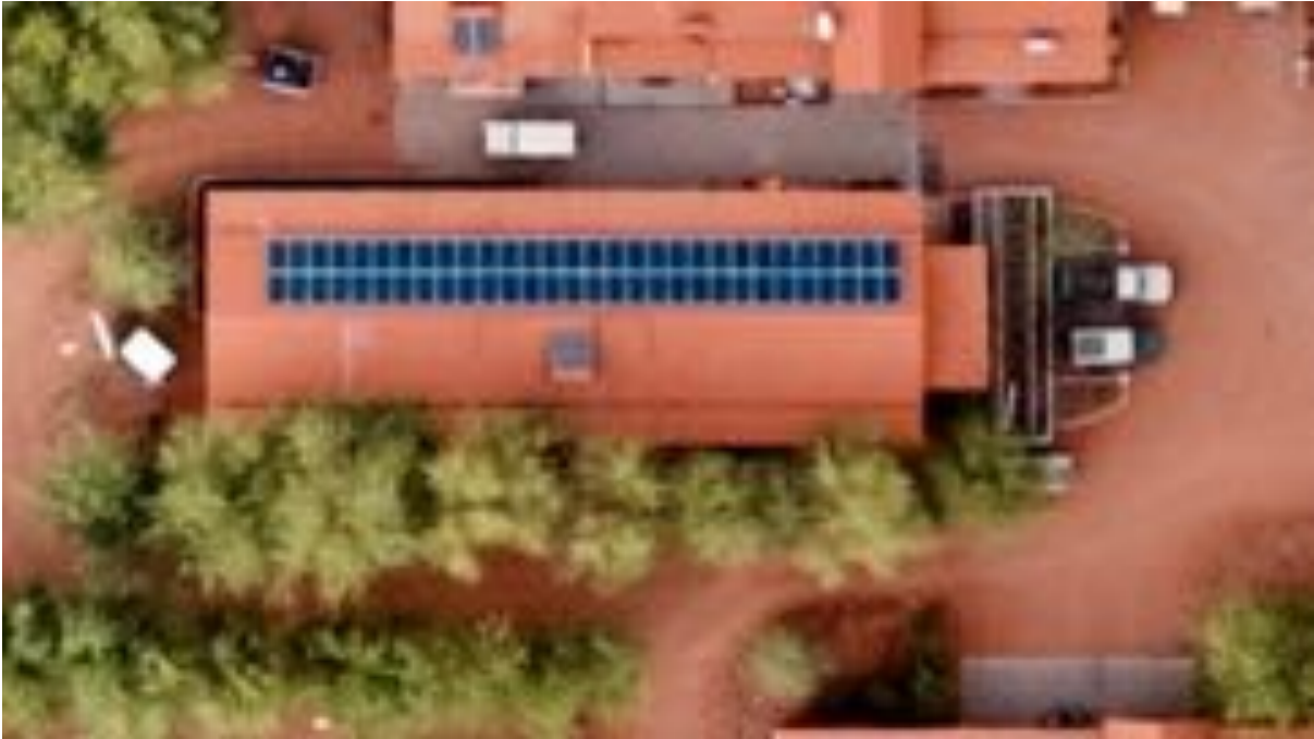
The new solar farm (17kW) positioned on the main stores and feeding into the Wolwedans grid when the sun shines
